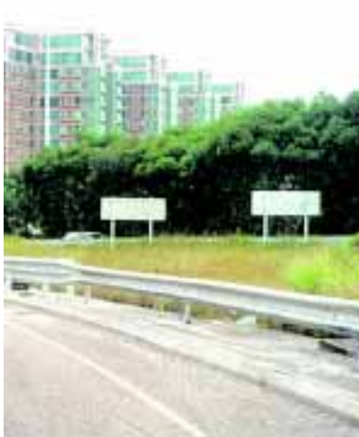
三波式防撞欄(天水圍朗天路)。 Thrie-beam safety barrier at Long Tin Road, Tin Shui Wai.
