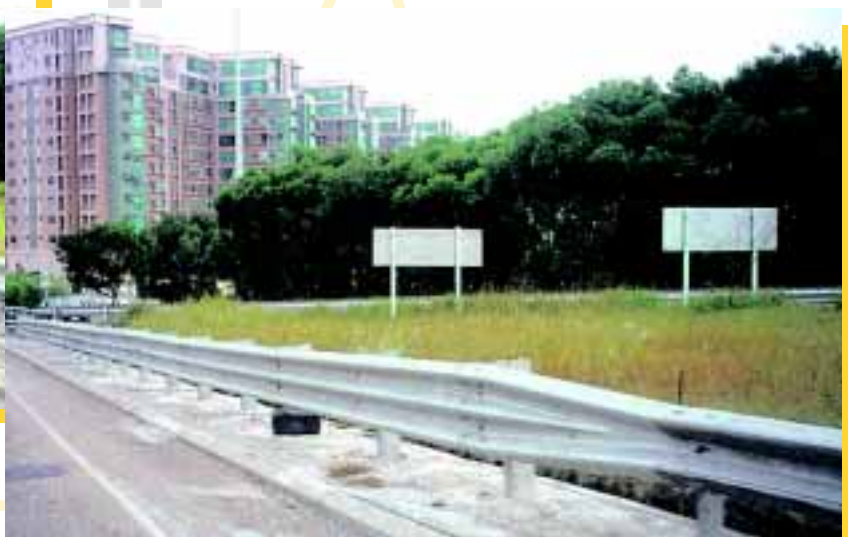
三波式防撞欄(天水圍朗天路)。 Thrie-beam safety barrier at Long Tin Road, Tin Shui Wai.
