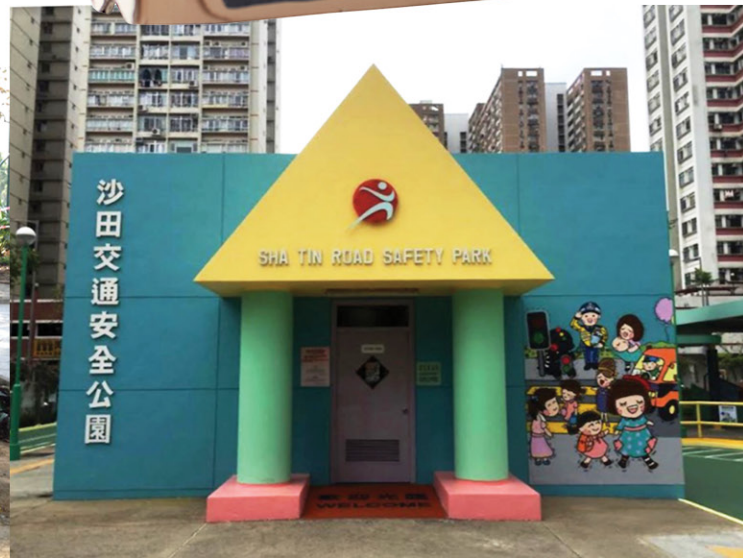
Sha Tin Road Safety Park 1 Kong Pui Street, Sha Tin | Enquiries: 2637 6303
